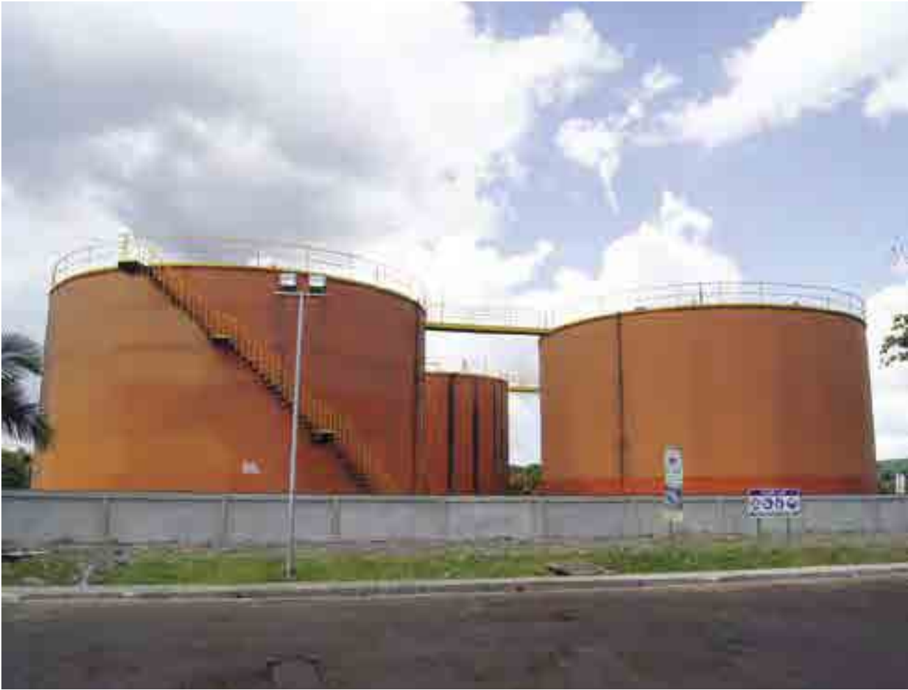
CPO Tanks at Mukah Palm Oil Mill
