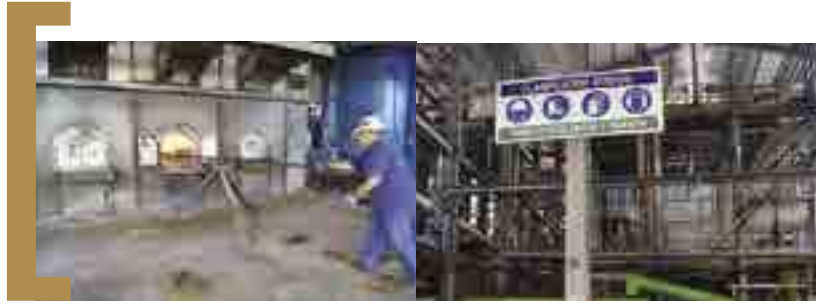
Raking of boiler fuel in the boiler furnace
