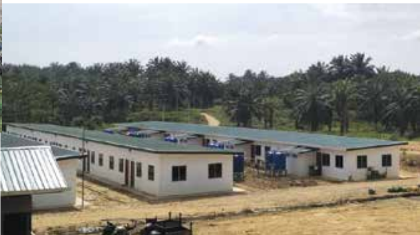
New workers' quarters
