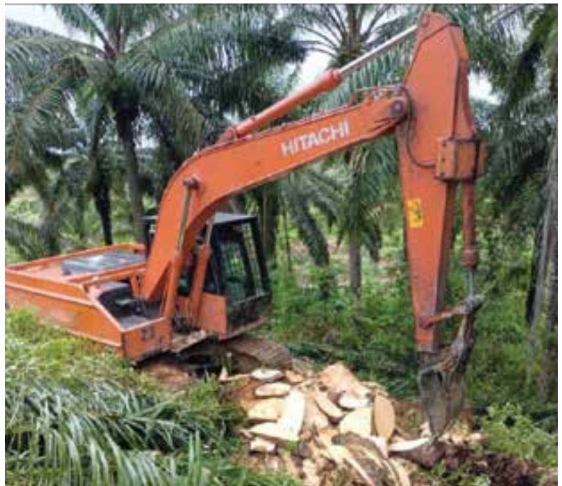
Chipping practice for replanting activities
