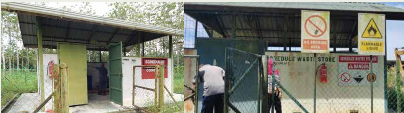
Scheduled Waste Store
